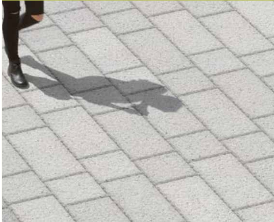
Public footpath to Trinity Road/ Partridge Way Permeable flags
