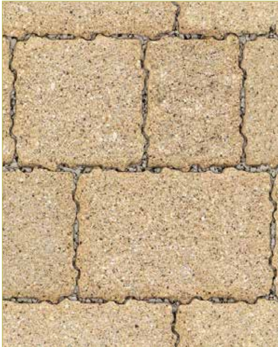
Disabled Bays Permeable blocks
