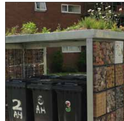
Green roof to bin store
