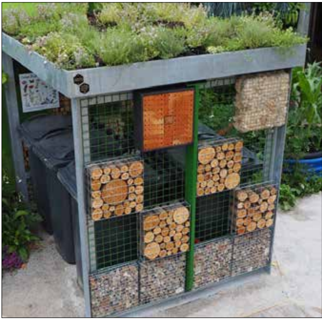
Bin store with green roof and invertebrate habitat
