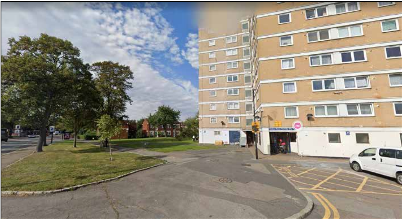
5.6 View of the entrance to Finsbury House
