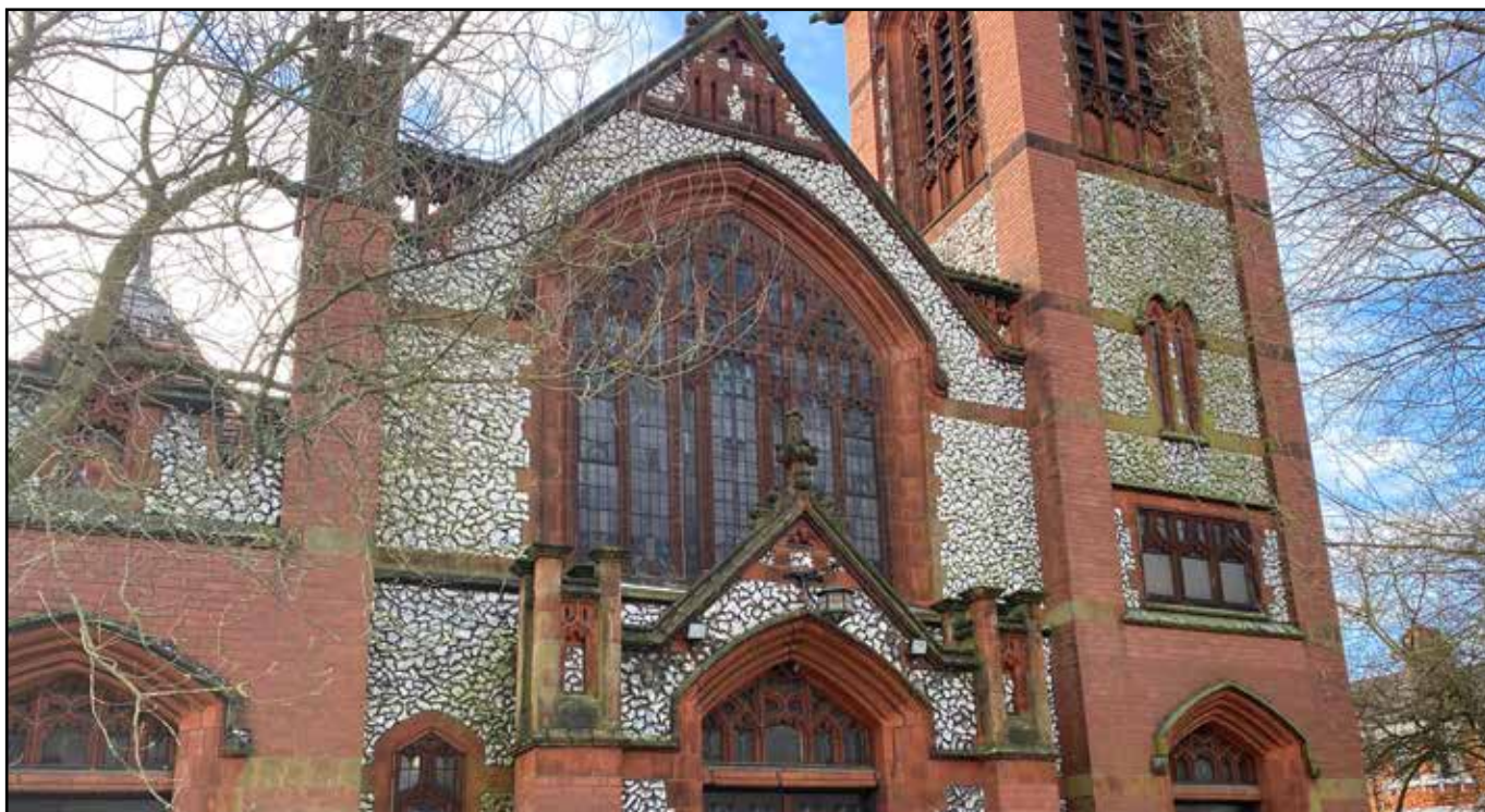
6.6 Braemar Avenue Church with white and grey flint detailing
