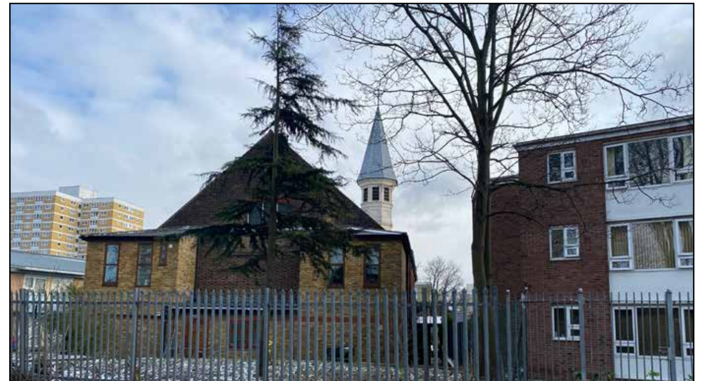
6.4 Rear view of St Barnabas church located on Finsbury Road in yellow brick with grey tiled spire
