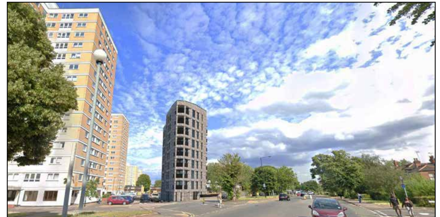
23.4 Nine-storey tower with single-storey plinth and enclosed balcony corner view
