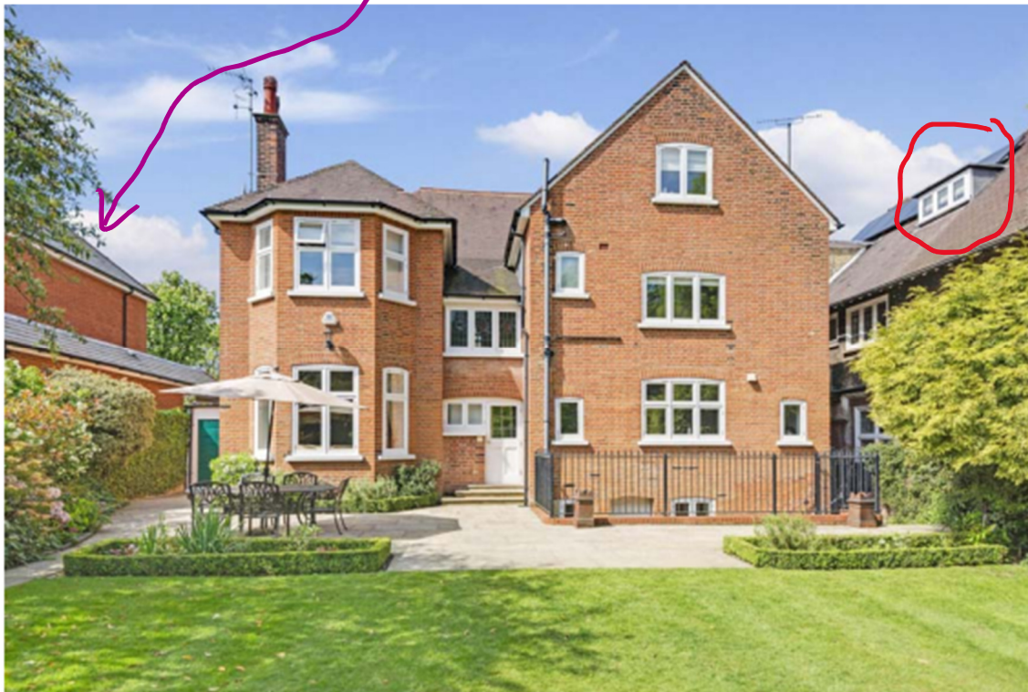
Photo 1 ( dormer window before works – it is about 1-2m away from the roof side ridge line; there was no direct view of our terrace; no window facing our property on No.18)
