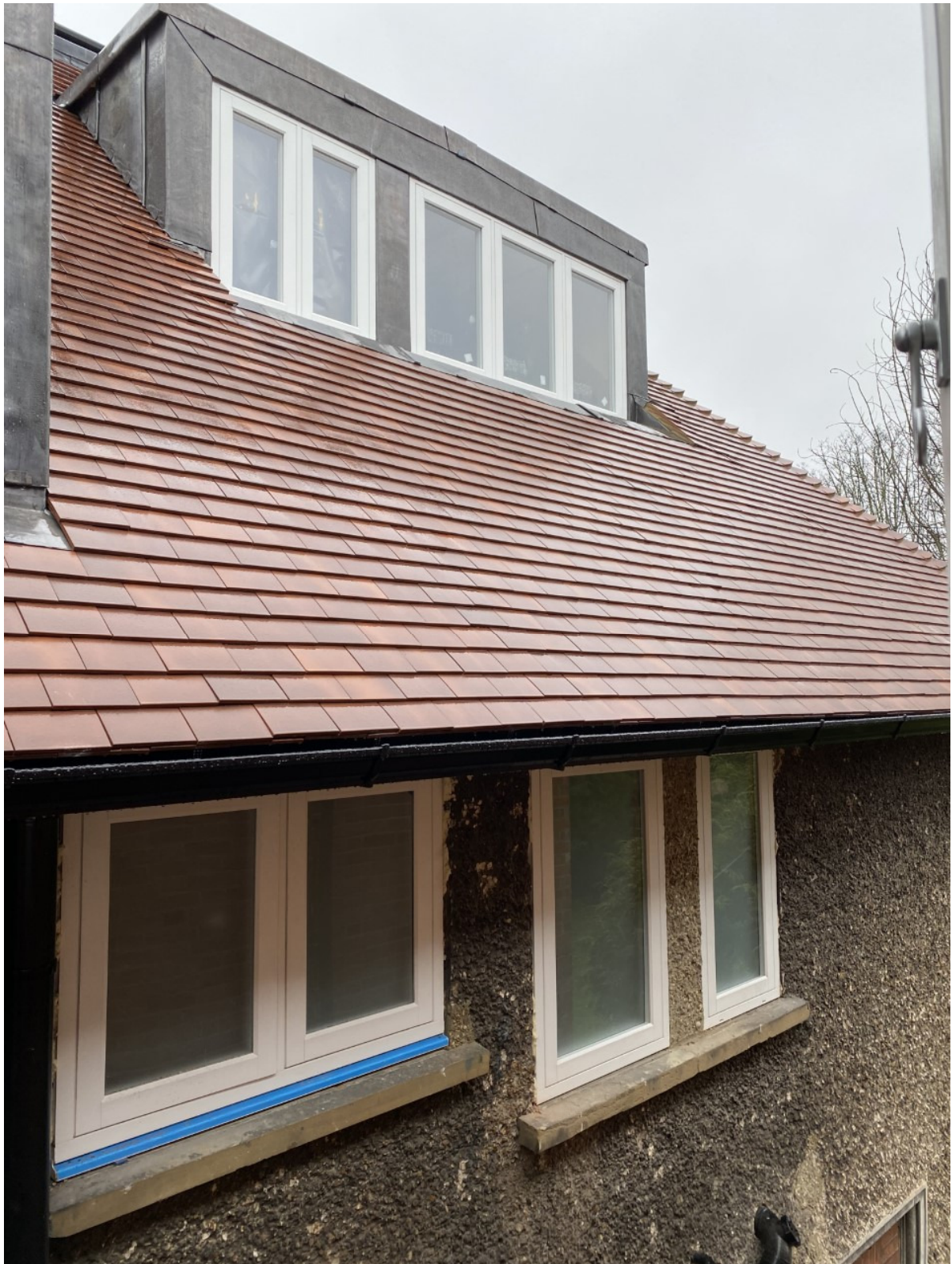
Photo 4 (side elevation windows that have been replaced with plain glass panels instead of lead latticing)
