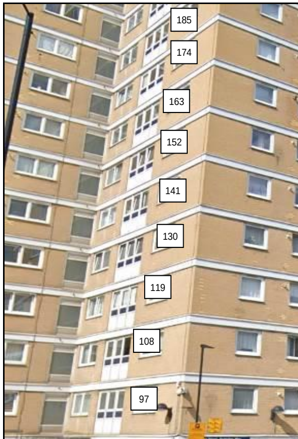
1 to 84 Finsbury House
