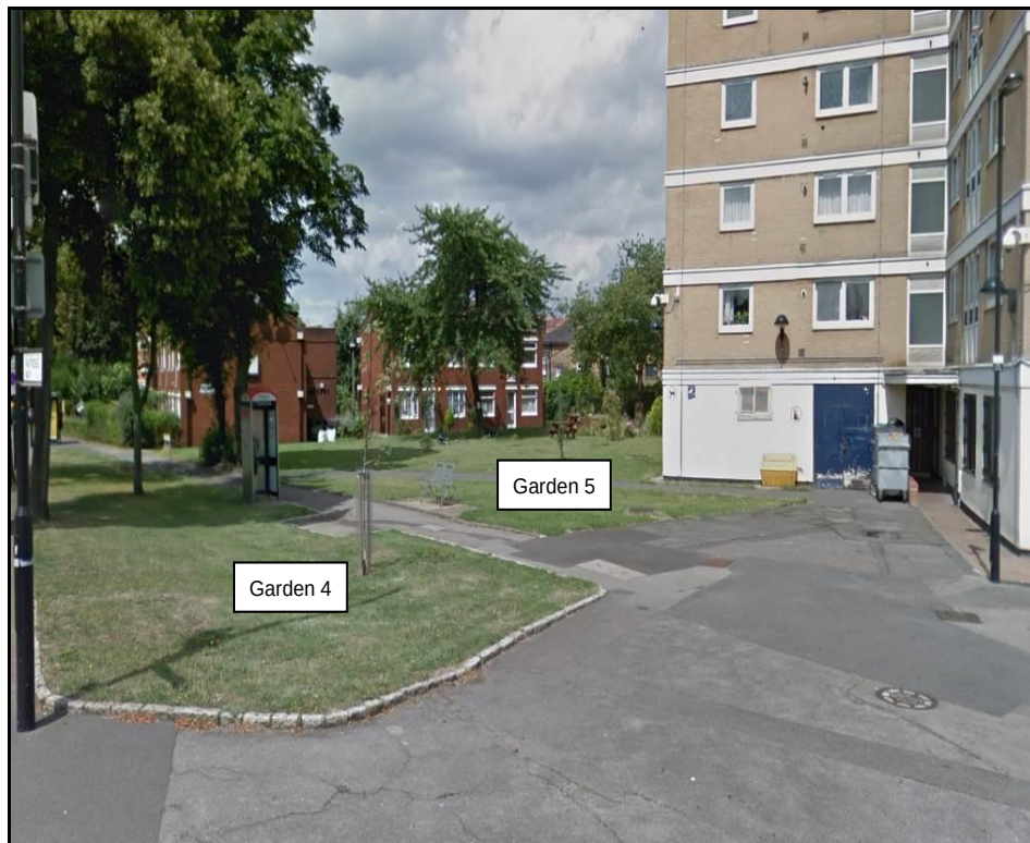
1 to 84 Finsbury House
