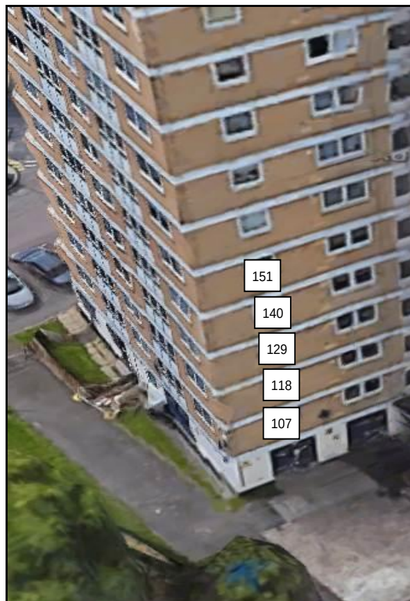
1 to 84 Finsbury House
