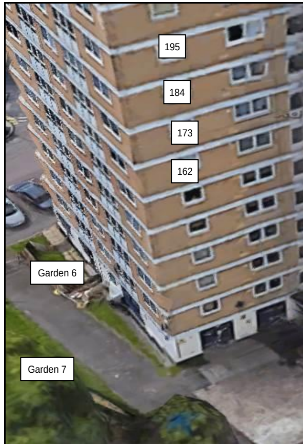
1 to 84 Finsbury House
