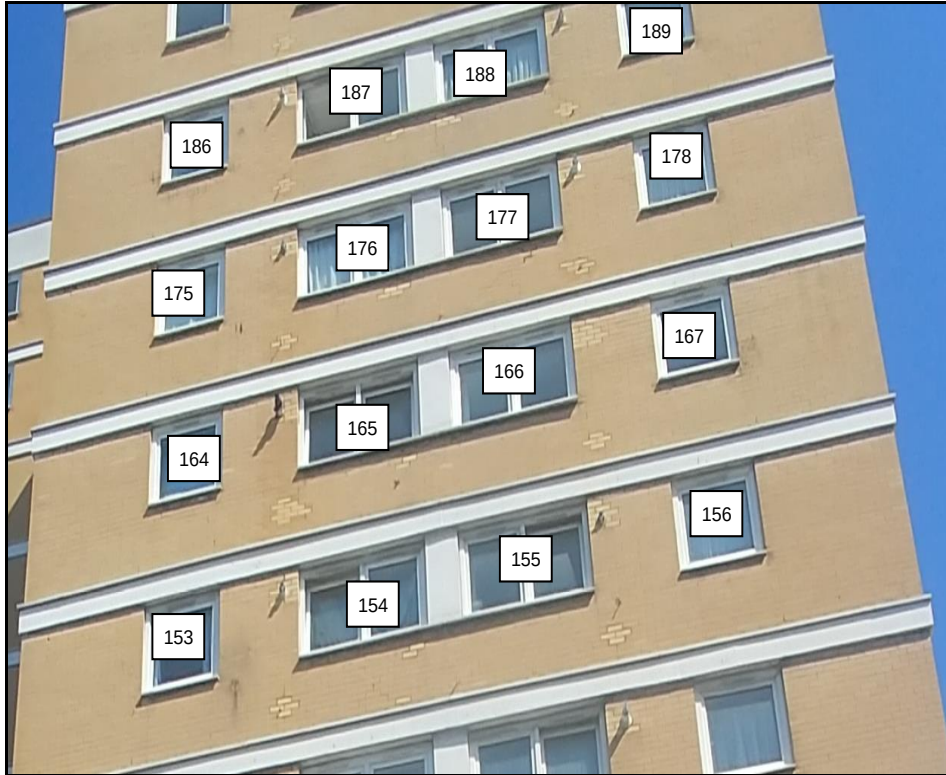
1 to 84 Finsbury House
