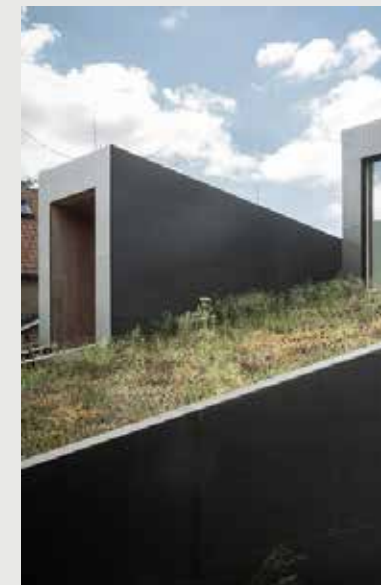
Angled green roofs
