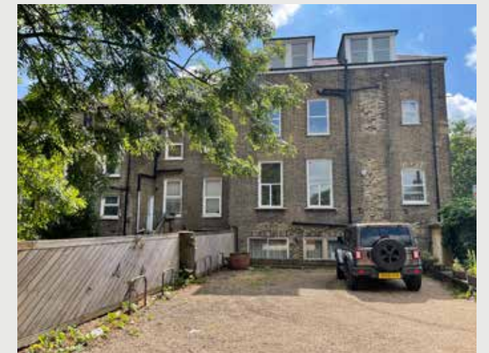
6. View towards southern boundary of site
