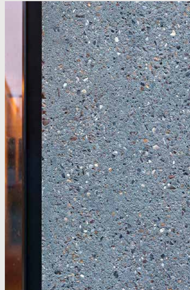
Textured precast lintels, entrances, copings
