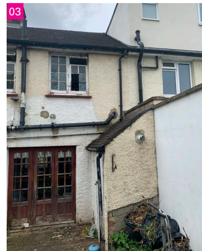
Rear of property showing neighbouring property number 8 extensions
