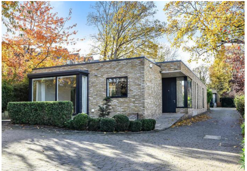
Existing building at No. 1 Olivers Row. Same bricks is going to be used for the proposed outbuilding. (view from north-east).
