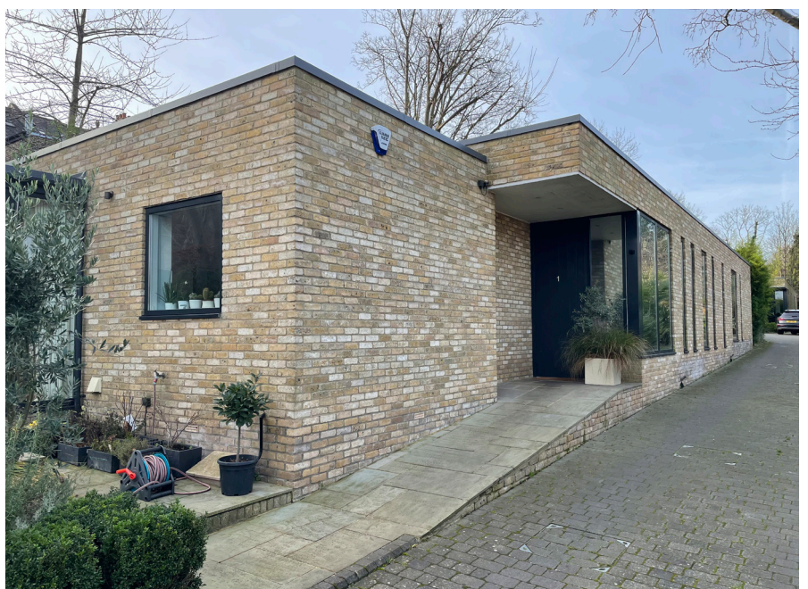
Existing building at No. 1 Olivers Row. Same bricks is going to be used for the proposed outbuilding. (view from north-east).
