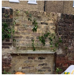
Existing front garden patch wall
