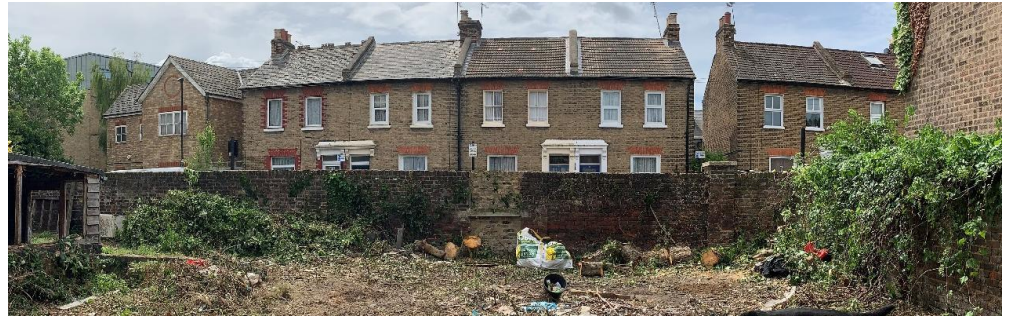
Existing front garden wall (Internal site facing)
