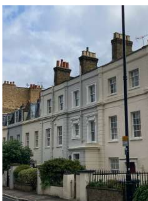
Figure 25. – Front façade no 46 – 38 (from right to left) indicating there are less pipes visible from their front façade
