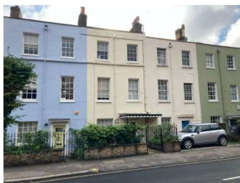
Figure 26. – Showing front façade of no 30 – 24 (from left to right), whose roofs are traditional butterfly roof
