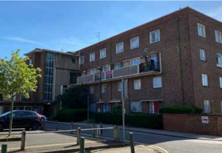
Existing facade treatment
