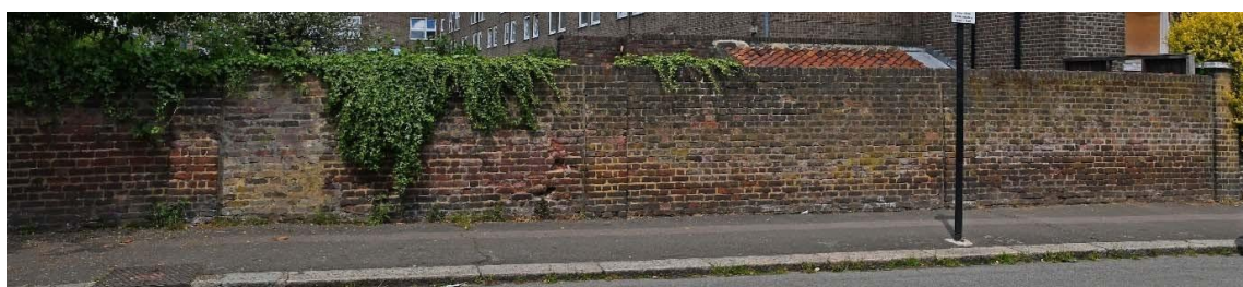
Figure 13. C19 roadside boundary wall (1). The blocked opening is towards the left.
