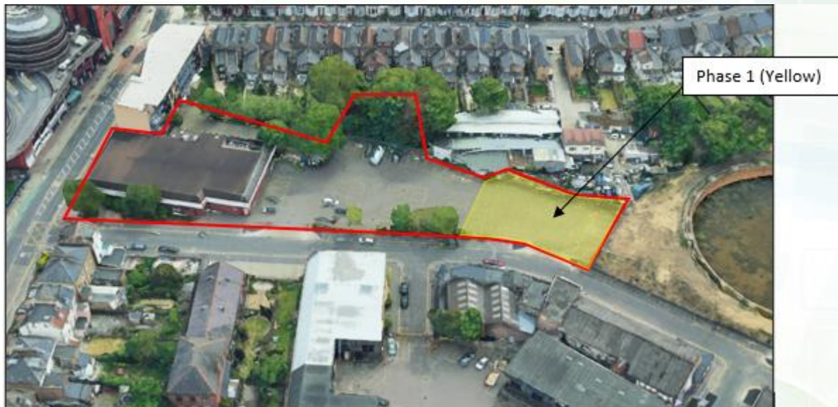
Figure 1: Aerial Image for the Site
