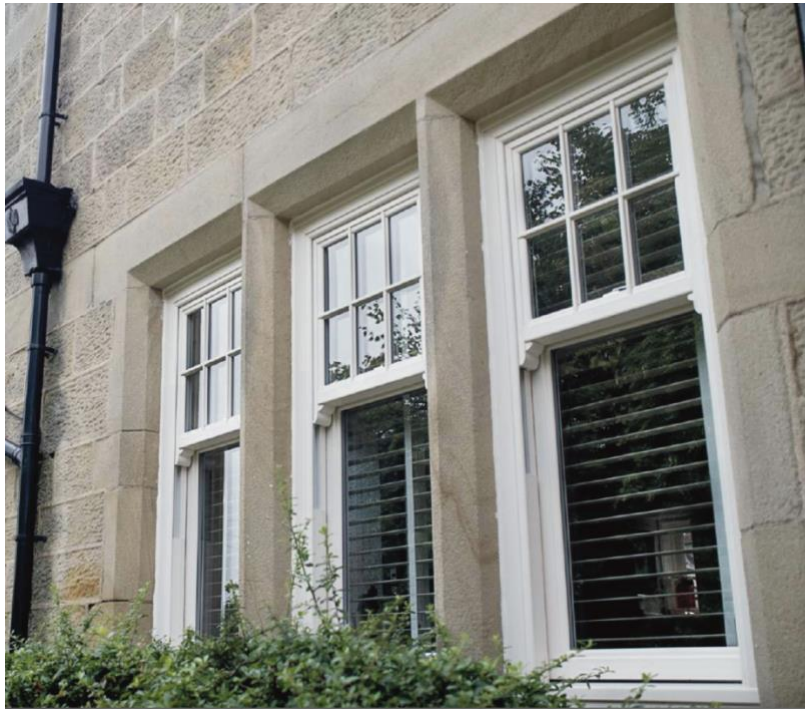
Photo showing new sash windows
