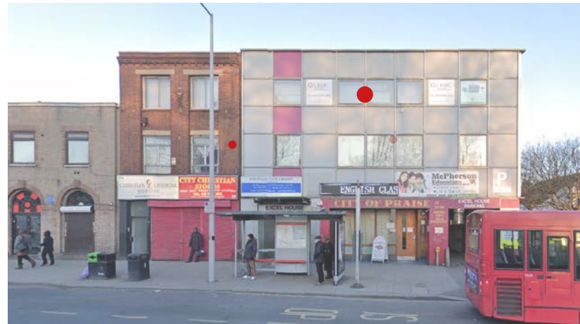
PRINCE REGENT LANE - STREET VIEW ● NO. 312 TOTTENHAM HIGH STREET
