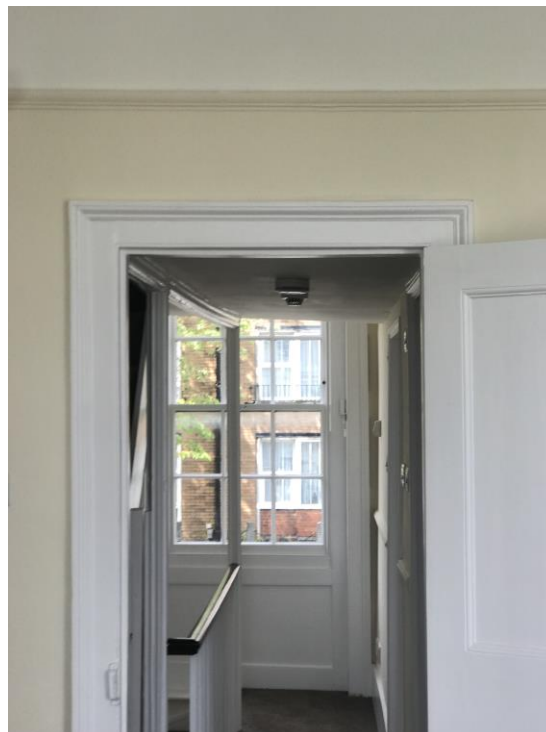
First Floor Props at edge of stair Supporting service tank enclosure
