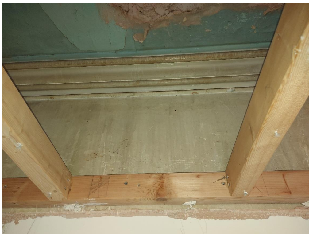
Figure 10: The timber inserted ceiling below the cornice in the second floor front room
