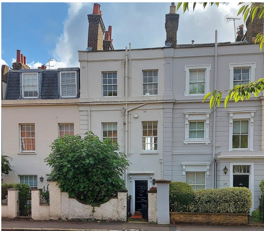
Figure.5: The street front of 42 Southwood Lane
