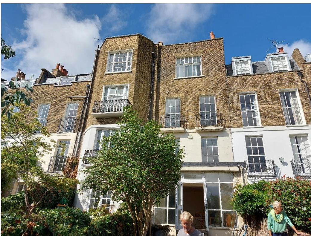
Figure 6: The rear elevation of number 42, to the right of the canted bay of number 40.
