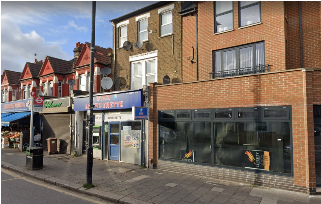
EXISTING FRONT ELEVATION PHOTO
