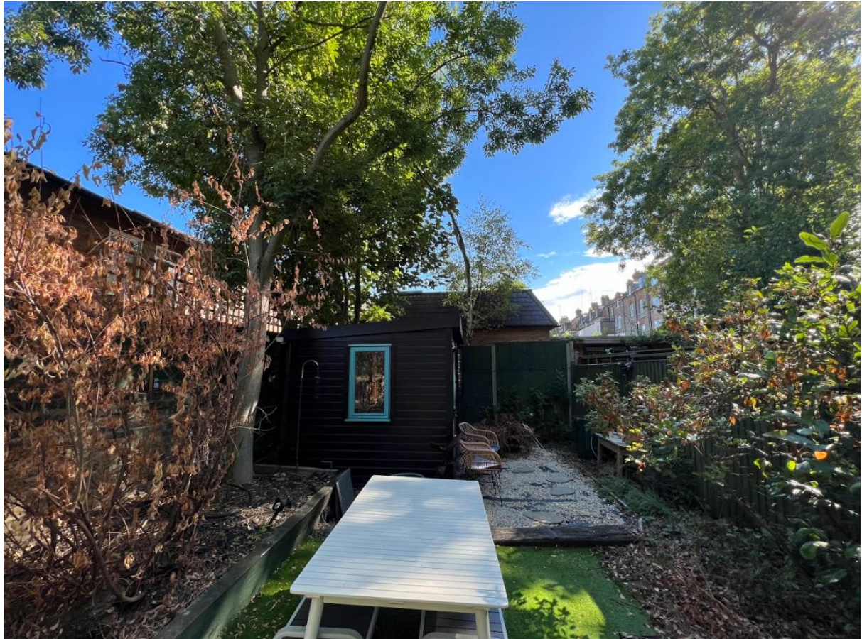
Existing timber building to be removed.
