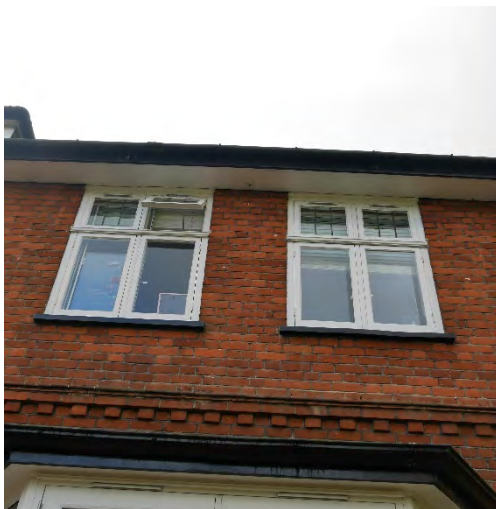
Figure 35: left; windows in the main part of the building, top lights are leaded but lower ones are not, right; over-sized and overly numerous windows in the side extension
