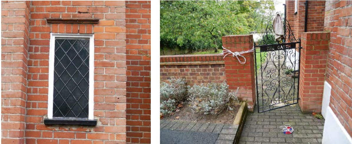
Figure 39: left; ground floor window, painted over, right; modern garden wall and gate dividing the front and rear of the property
