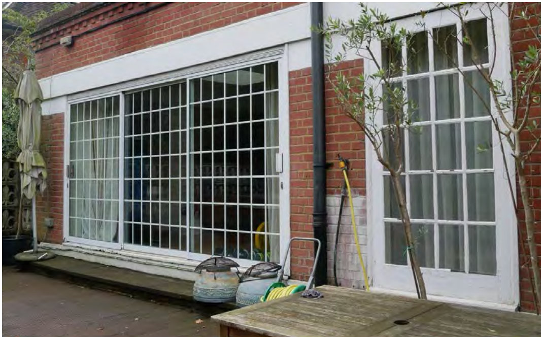
Figure 29: Sliding doors to the garage extension (now a gym) with modern, double-glazed uPVC sliding doors installed into the original timber frames. Glazing bars are false "Georgian Bars", set between the two panes.
