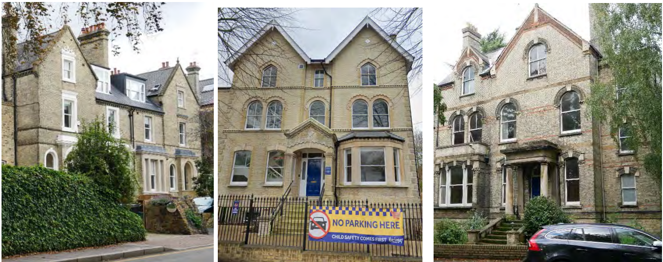
Figure 18: Victorian Buildings on Bishop'swood Road (left and centre) and Broadlands Road (right), the central building is in use as part of Highgate Pre-preparatory School
