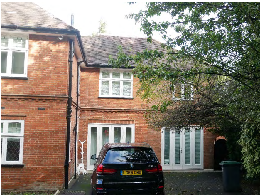
Figure 33: View of the extension to the right showing two sets of double French doors with parliament hinges
