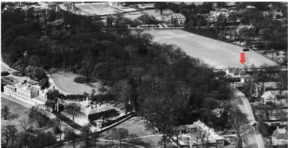
Figure 6: The subject buildings are seen in the 1938 aerial photograph and their planform bears resemblance to their current form. The half timbered protruding gable, Arts & crafts windows, steep pitched roof and chimneys are seen in this view.
