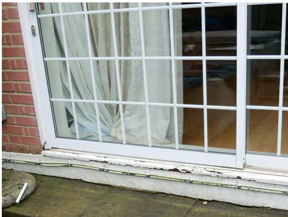
Figure 29: Sliding doors to the garage extension (now a gym) with modern, double-glazed uPVC sliding doors installed into the original timber frames. Glazing bars are false "Georgian Bars", set between the two panes.
