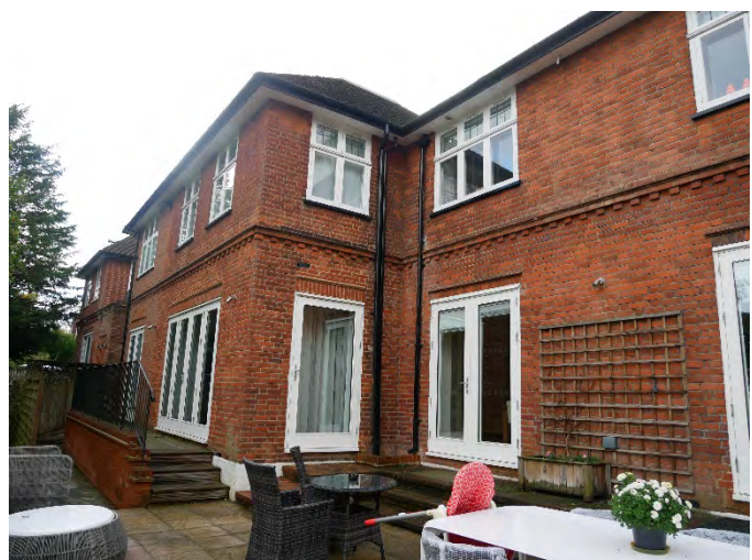
Figure 35: left; windows in the main part of the building, top lights are leaded but lower ones are not, right; over-sized and overly numerous windows in the side extension
