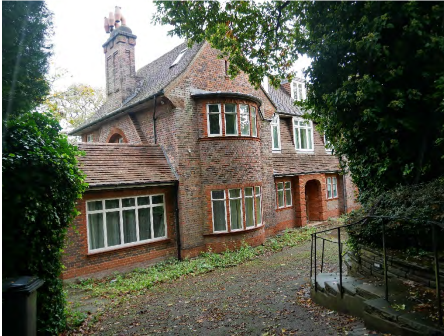
Figure 16: 42 Hampstead Lane 'Oakleigh', approved for demolition in 2017 (HGY/2017/1710)
