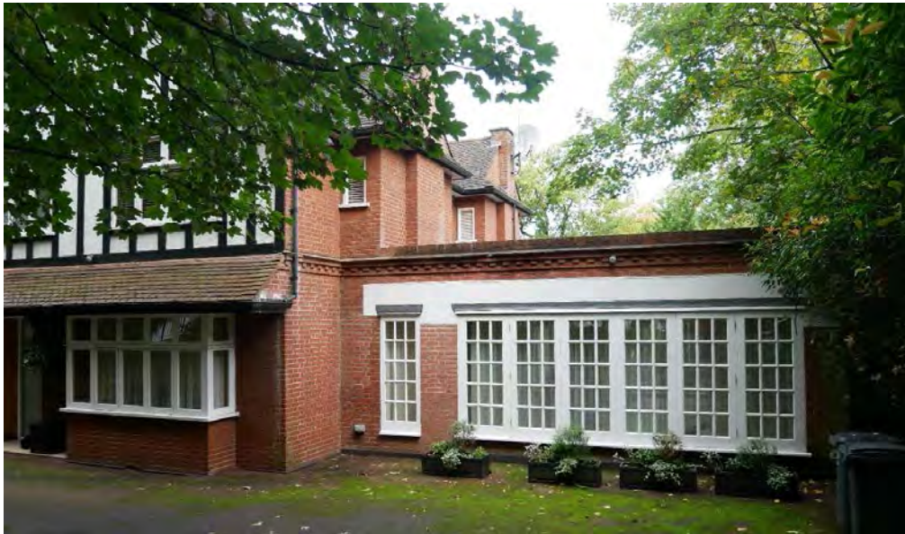
Figure 24: Single-storey extension to the east of the building, formerly a garage, believed to date from 1990s.
