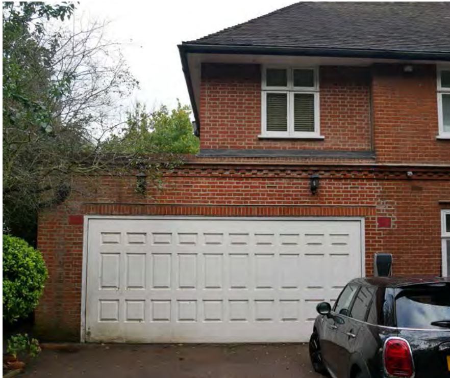
Figure 23: Garage extension which dates in part from 1972 and 1988 although thought to have been re-pointed more recently. First floor, recessed extension above was proposed and executed in 1998, HGY: 056960, (following the 1988 application HGY: 46267)
