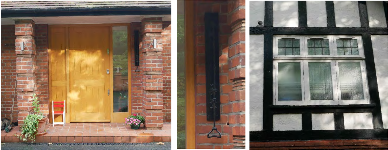
Figure 32: left; inappropriate front door with pillars that features articulated quoins, centre; authentic bell-pull, right; obscured glass in the right hand window of the two at first floor in the front gable
