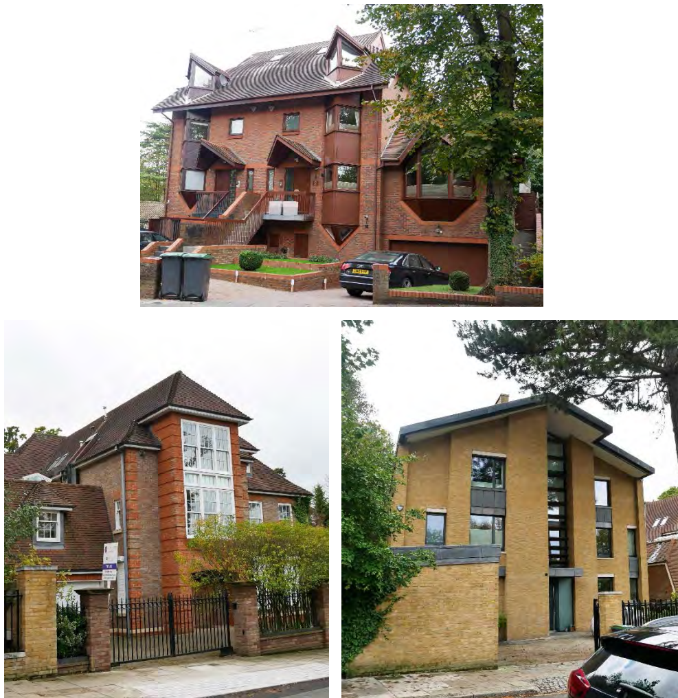
Figure 20: Modern buildings of a variant style on Denewood road, some reference Arts and Crafts and neo-Georgian features, whilst others represent a greater departure, referencing only the pitched roofs and overhanging eaves. These are all examples of buildings which extend three or four storeys, more akin to the Victorian townhouse form on Bishop'swood Road.
