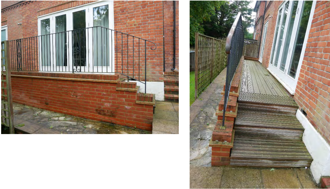
Figure 38: modern, elevated walkway with decking adjoining side extension
