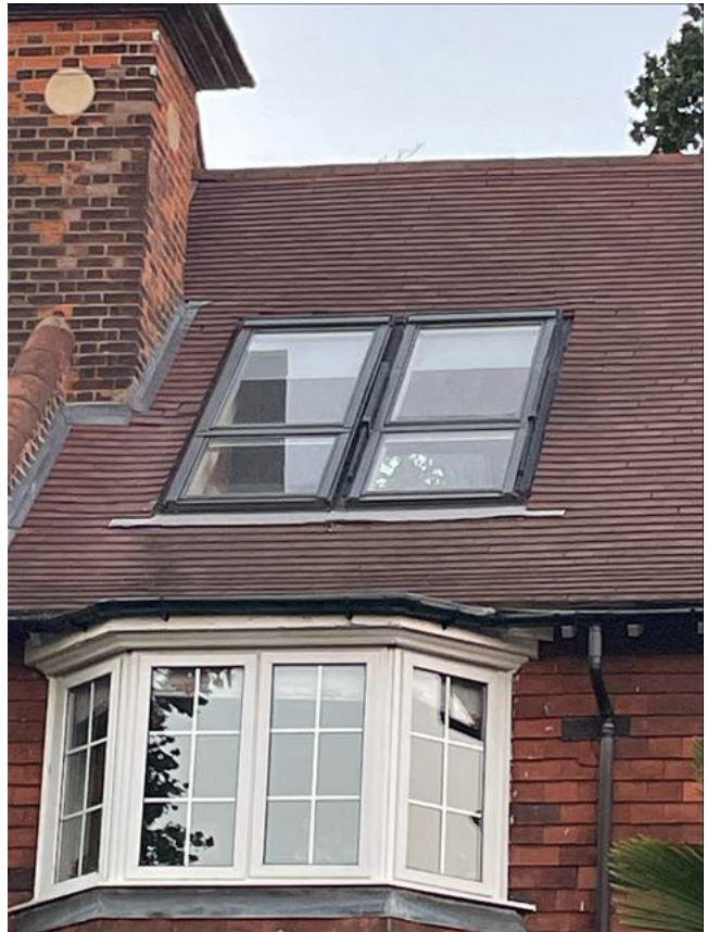
Zoom View, 2 x Skylight at the front elevation
