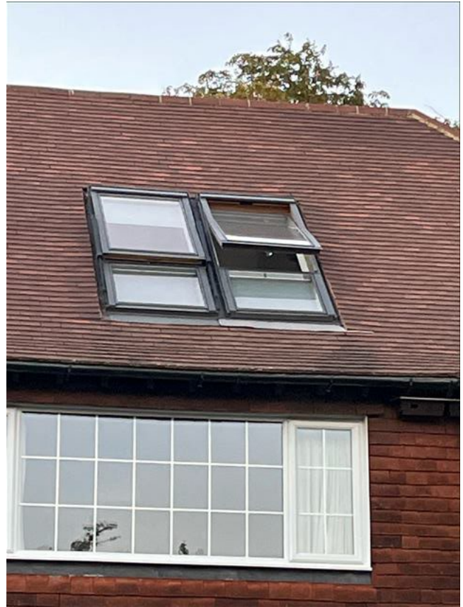
Zoom View, 2 x Skylight at the front elevation
