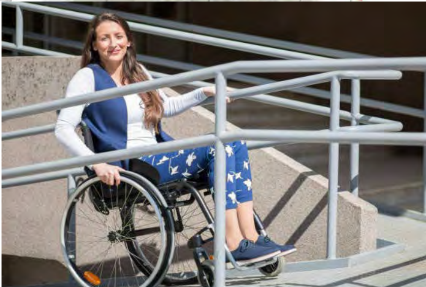
Ramp with 1:20 gradient
