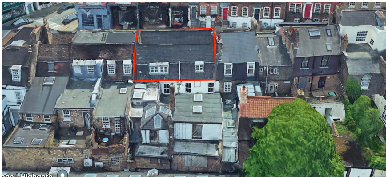
Figure 2. Flat C, 32/34 Highgate High Street (rear elevation)
