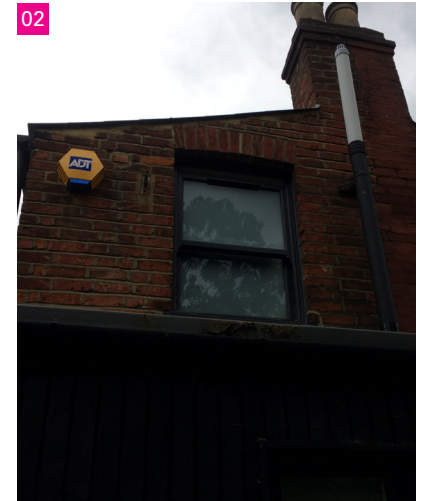
Existing rear first floor outrigger
