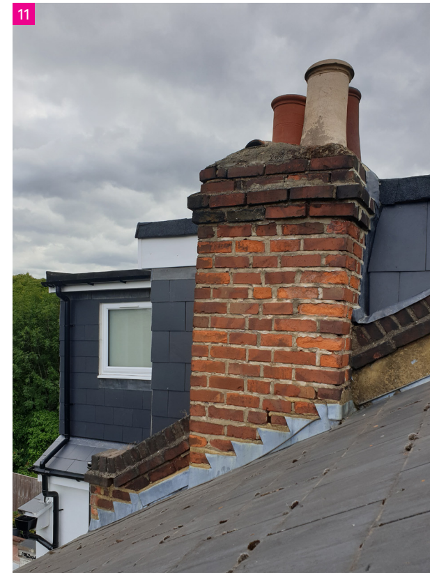
50 Seaford Road showing existing gable to be raised to create appropriate fire barrier between neighbouring loft extensions
