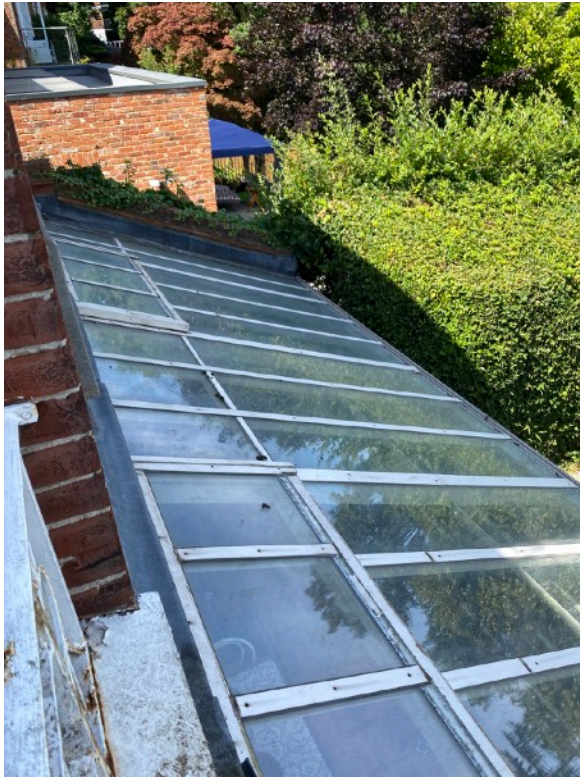
Conservatory Roof and View of No.65's Extension.
