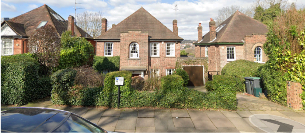
Gap between No.73 and 75. (Google Streetview).
