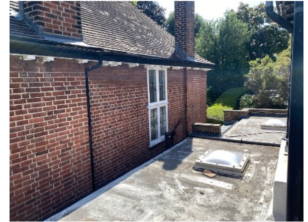
Roof of Existing Flat Roof to Side of No.67 and Flank Wall of No.69 with Window to Stairwell.
