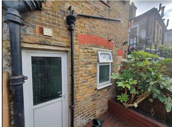
BELOW: Rear elevation 203 Gladstone Ave
