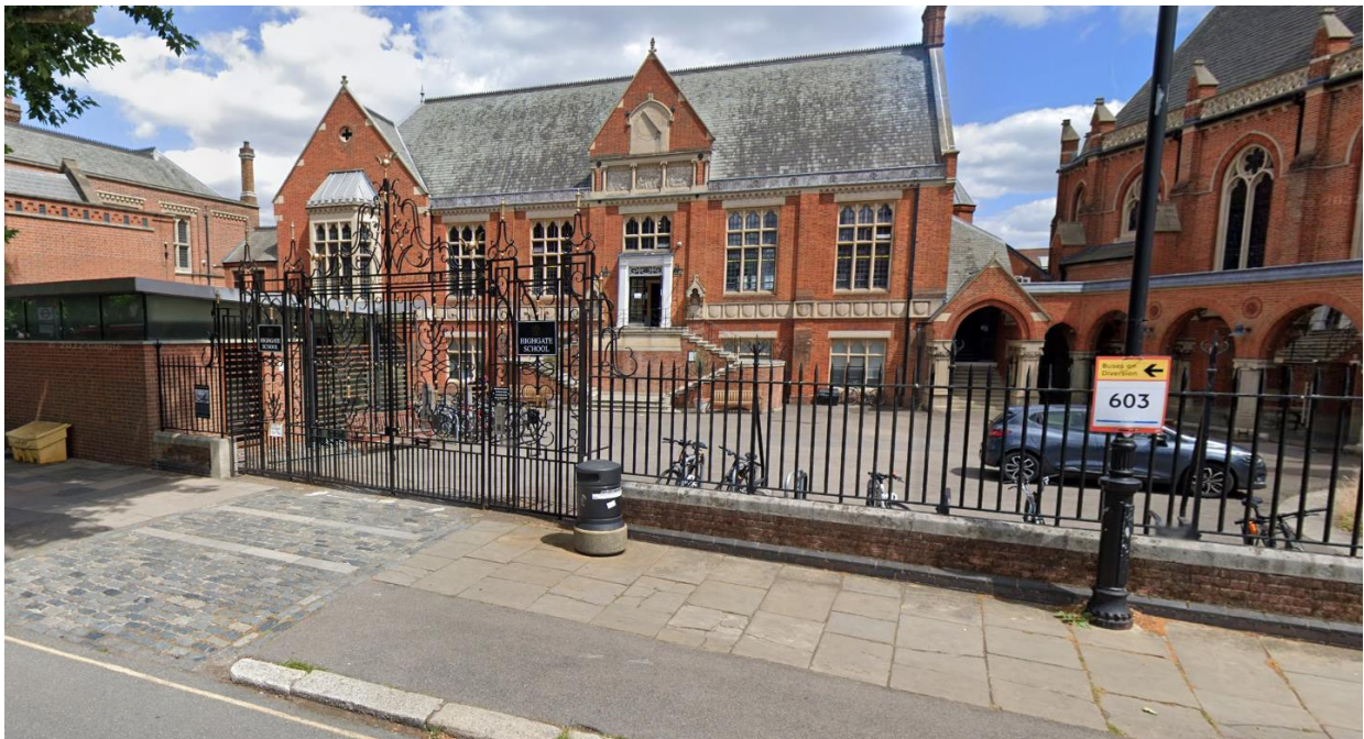
001 – Boundary railings prior to the impact damage
