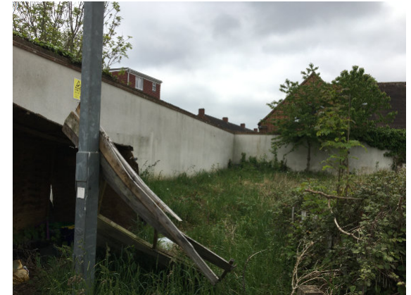
Boundary wall to the housing on White hart Lane.
