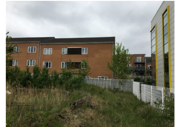
Housing to the North overlooking the site.
