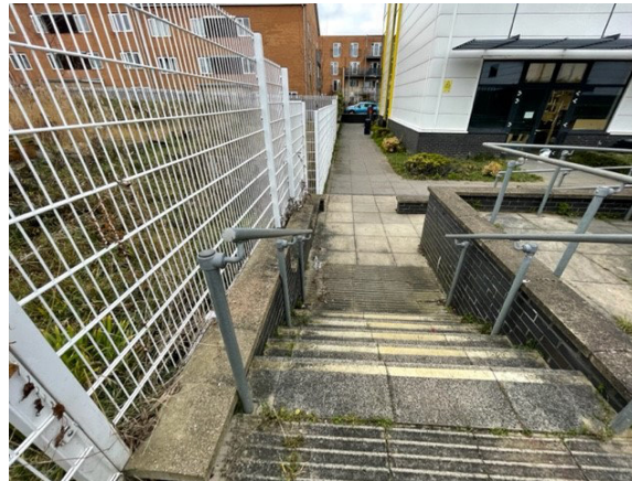
Existing steps and ramp to site
