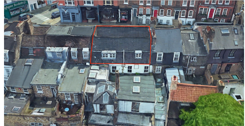
Aerial: Rear of house
