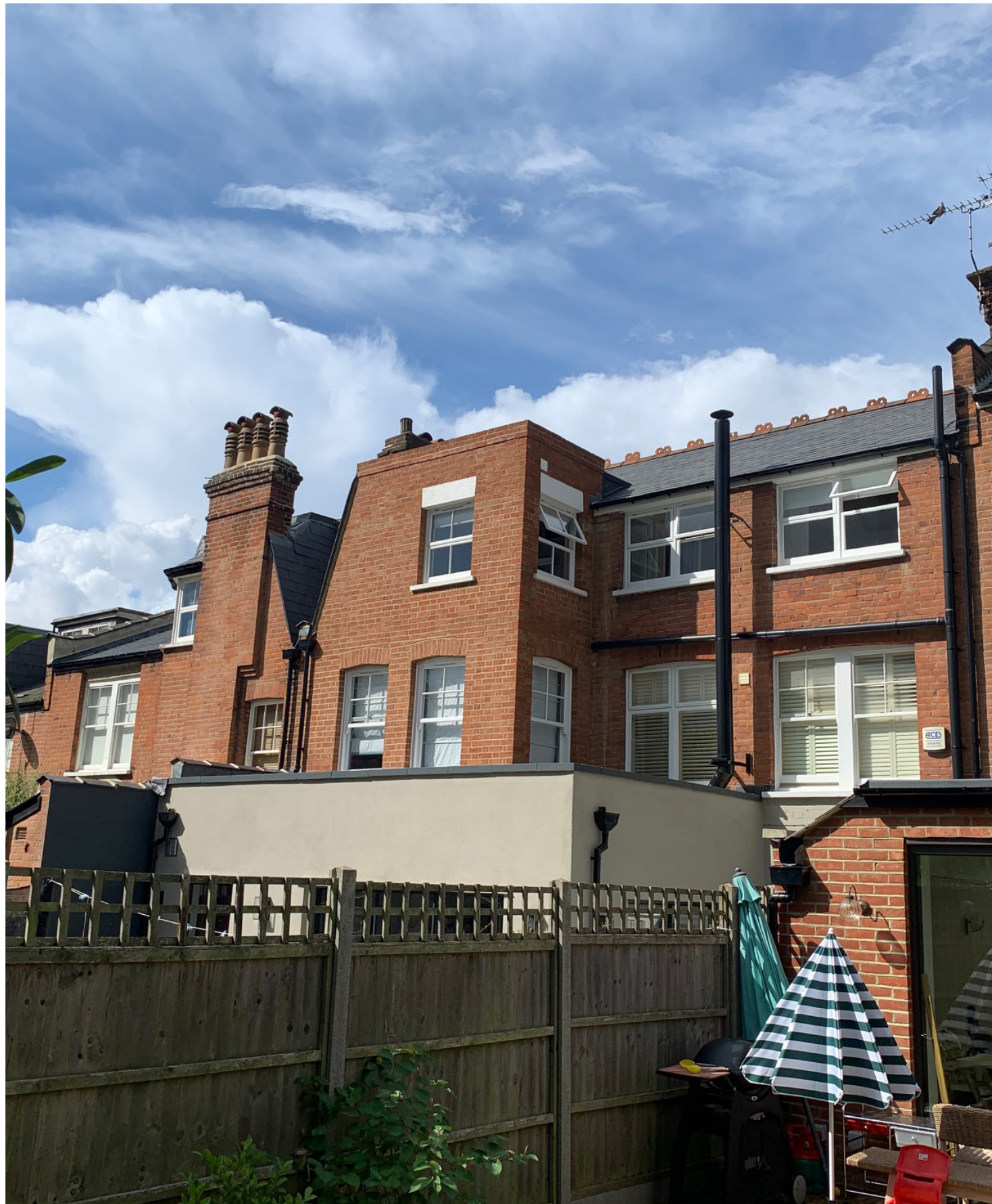
5. Existing neighbouring properties to left (viewed from garden).
