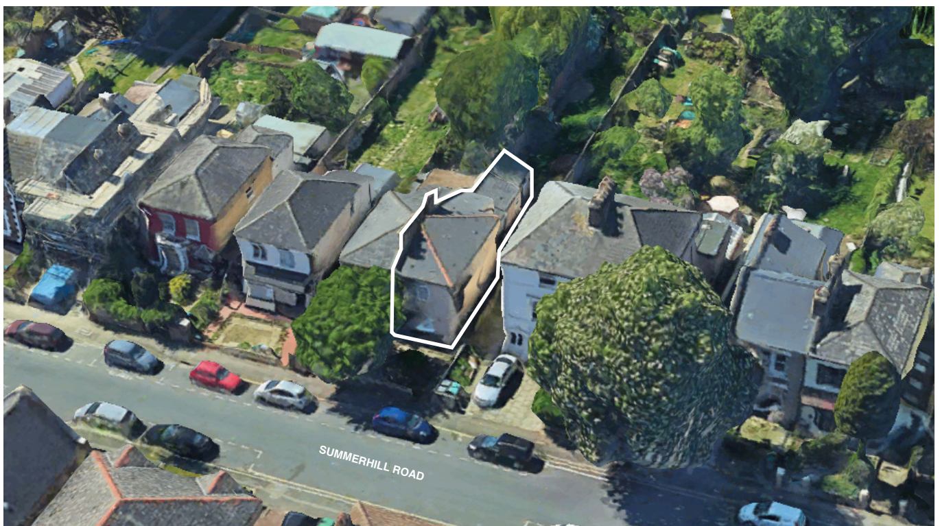
Aerial view facing south, site outlined in white.
