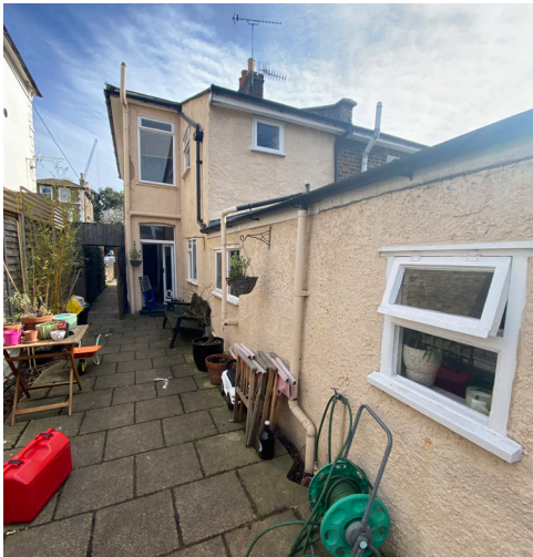
4. Photo of the existing rear outrigger.
