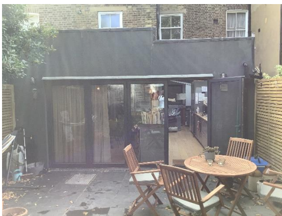
Rear elevation of main property
