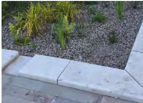
Kerb upstands with flush kerbs to allow water through around rain gardens
