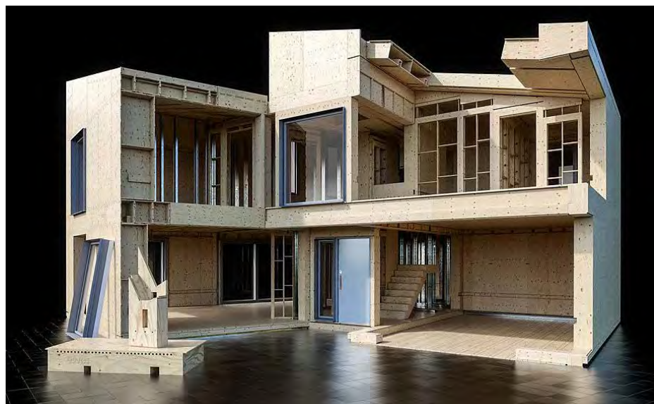
An example of Modern Methods of Construction, the Facit Chasis system by Facit House
