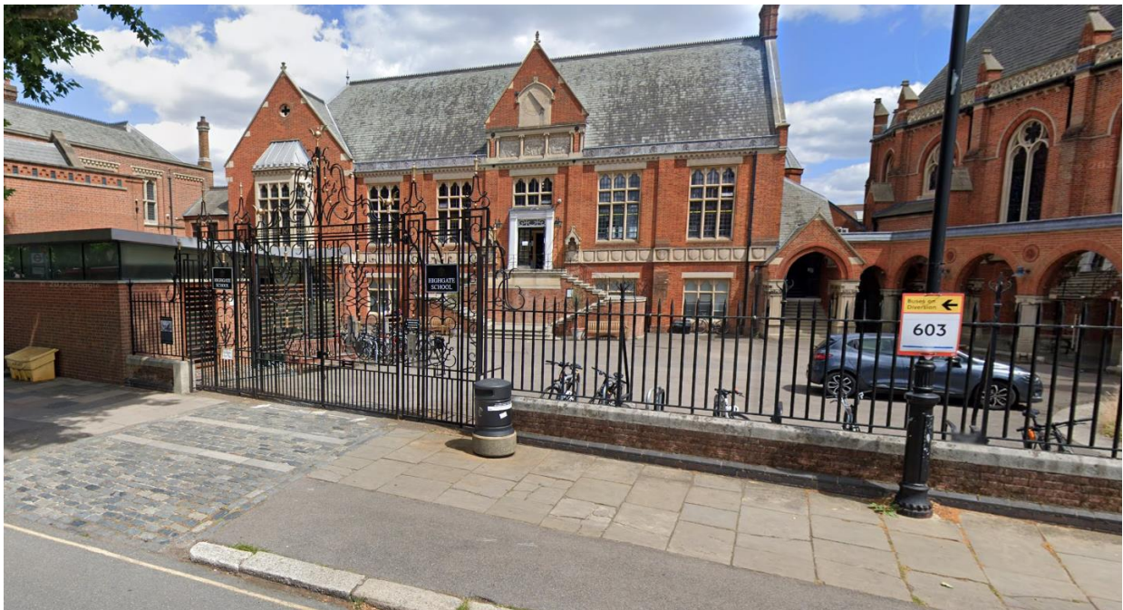
001 – Boundary railings prior to the impact damage
