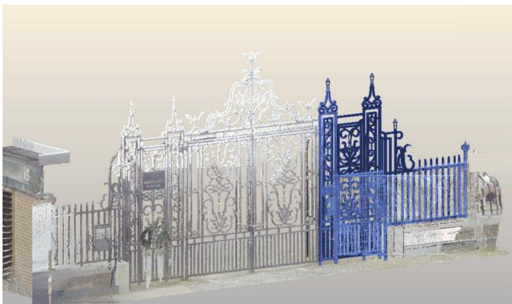
005 – 3D scan showing the damaged metalwork in blue
