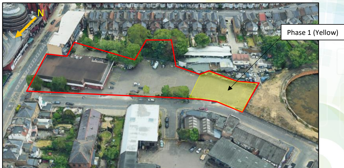
Figure 1: Aerial Image for the Site (approximate site boundary in red), PHASE 1 in YELLOW
