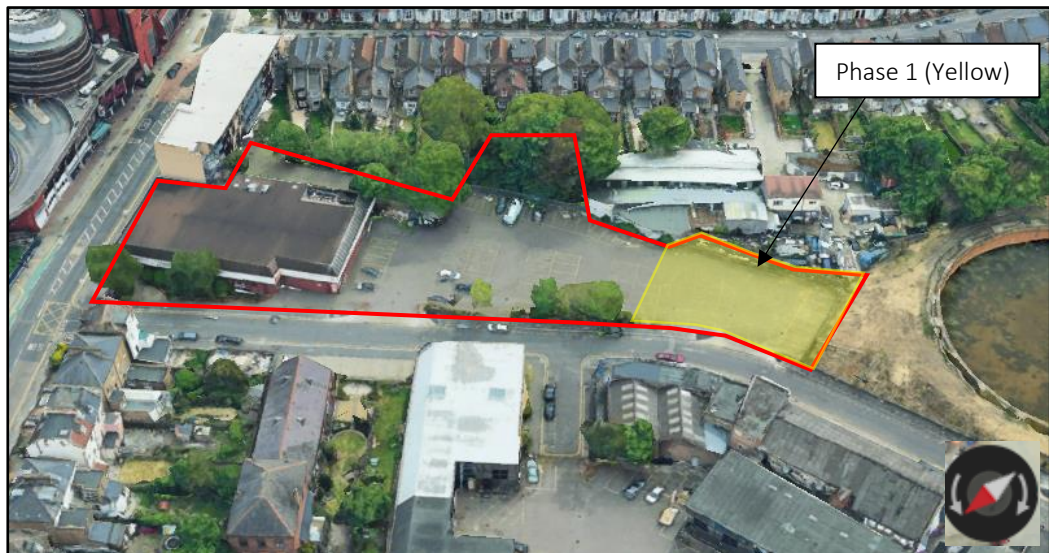
Figure 1: Aerial Image for the Site (full site boundary in red)
