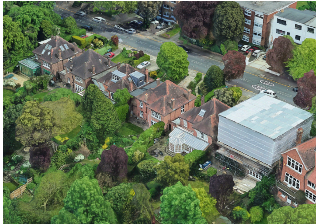
Aerial image from Google Earth showing development of the group of six houses from the rear. The scaffolding is No.65 undergoing a rear extension and roof extensions.
