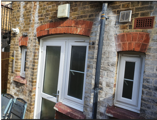
A photograph of a brick building exterior. On the left is a white door with a large glass panel. To the right of the door is a small, white-framed window. A large, leafy green plant in a wooden planter sits on a wooden deck in the foreground. A black downspout runs vertically along the brick wall. In the background, another brick building with a balcony is visible.
