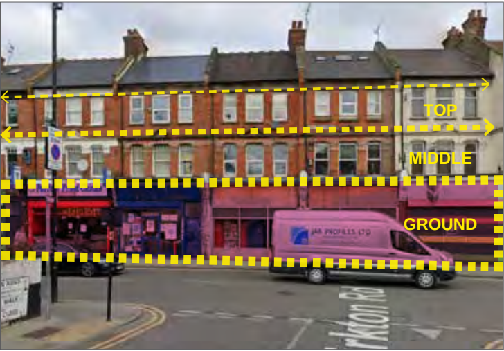
Existing shop front terraces along West Green Road
