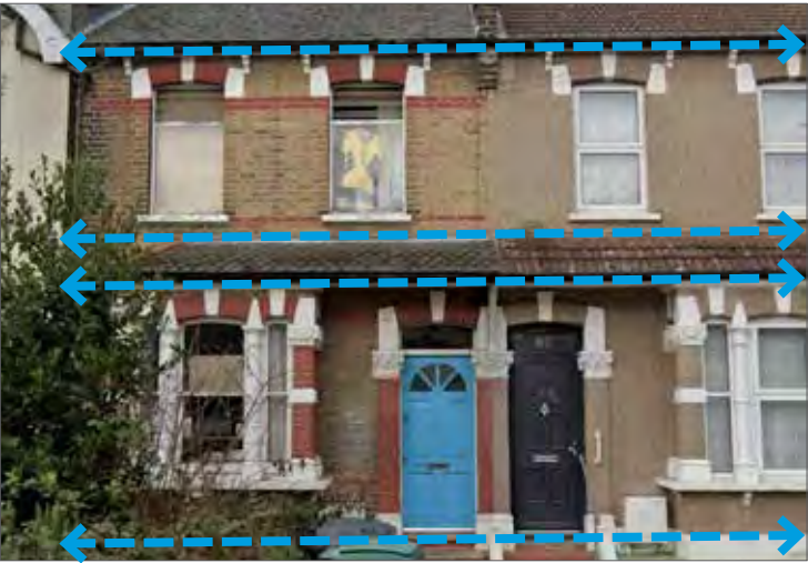
Existing terrace facade of No. 81/83 Kirkton Rd (west)
