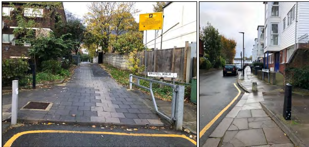
Photographs 1 and 2: Existing Footways
