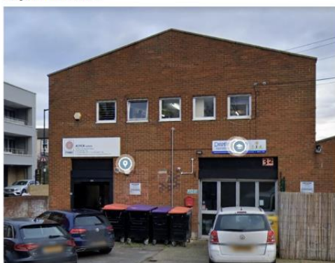
The existing site
