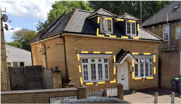
Figure 10: 8 Hornsey Park Road
