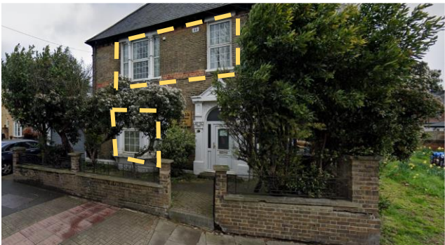
Figure 11: 10 Hornsey Park Road
