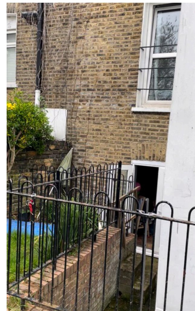
Garden: Existing garden is higher than lower ground floor flat. Existing retaining wall creates poor access from the flat to the garden and creates long shadows internally.
