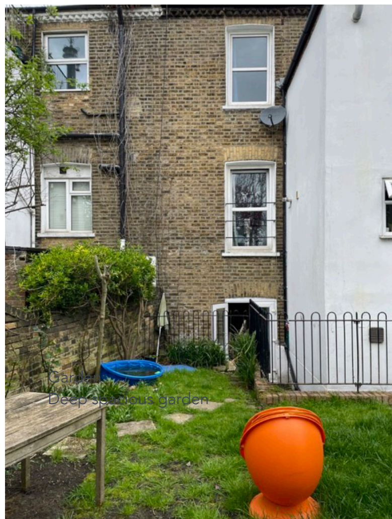
Garden: Existing garden is higher than lower ground floor flat. Existing retaining wall creates poor access from the flat to the garden and creates long shadows internally.
