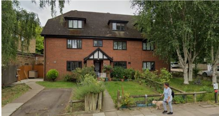
2. Casement windows at 1 Grange Road facing View Road
