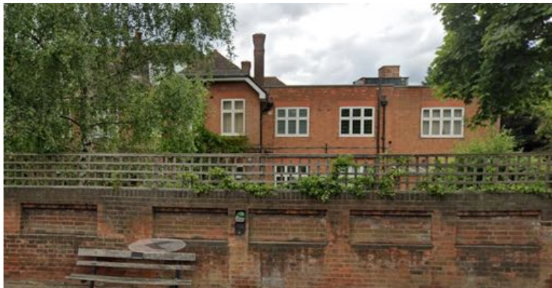
3. Casement windows at 1 View Road
