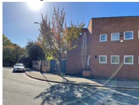
Building NE corner
