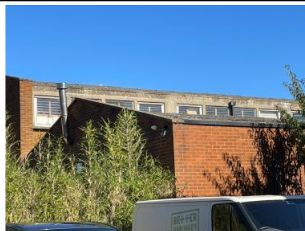
Roofs of building looking NE
