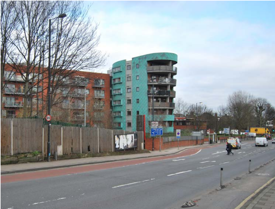
VIEW 2 LOOKING EAST FROM TURNPIKE LANE
