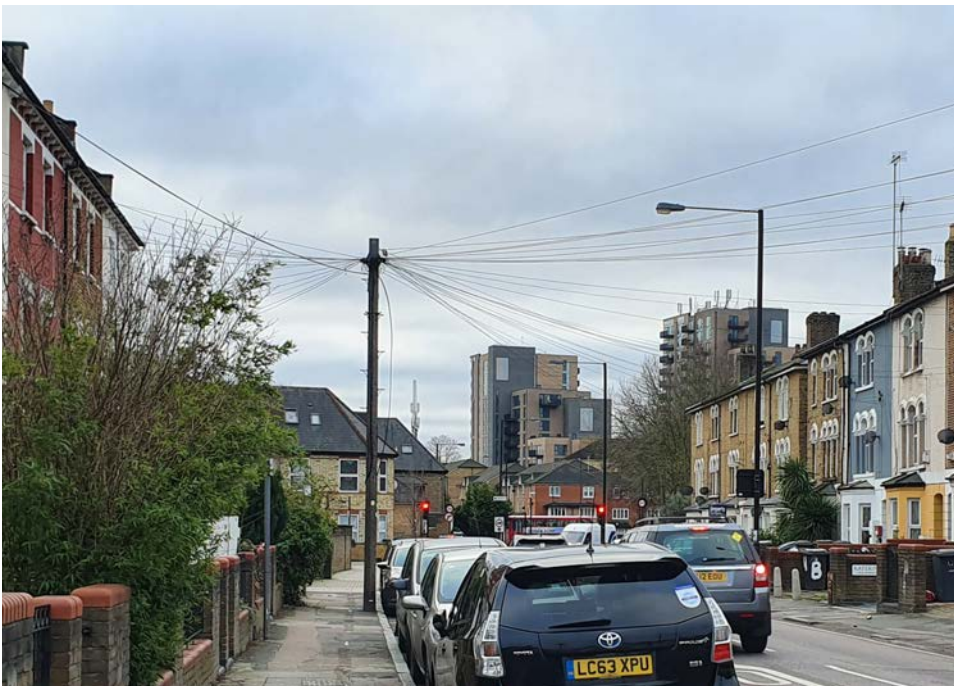
VIEW 4 LOOKING SOUTH FROM HORNSEY PARK ROAD
