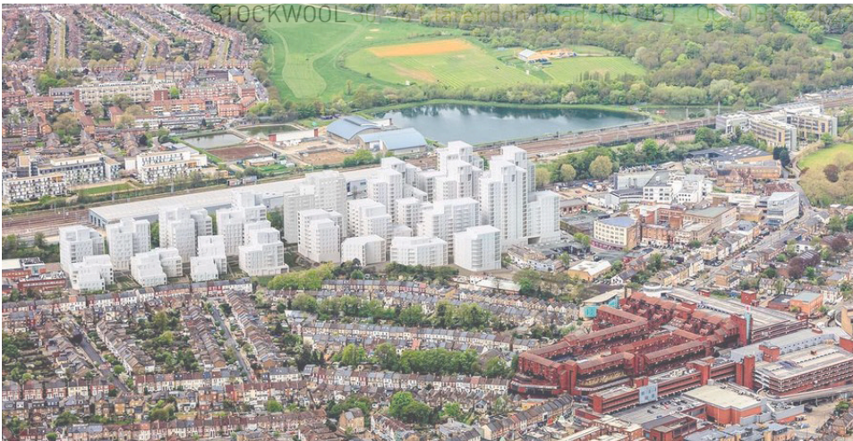
GAS WORKS MASTERPLAN UNDER CONSTRUCTION
