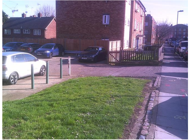
Main entrance, view south from Boyton Road.
