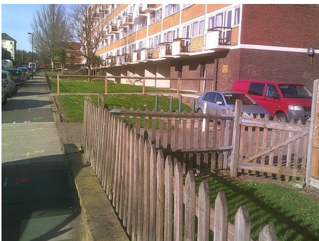
Soft landscaping on the south-west corner, view north.
