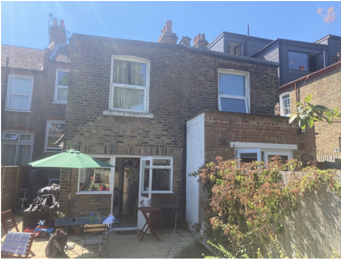
Rear view of kitchen windows and doors, with adjacent extension at number 32 Mattison Road
