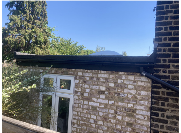
Side view of neighbouring extension at number 36 Mattison Road
