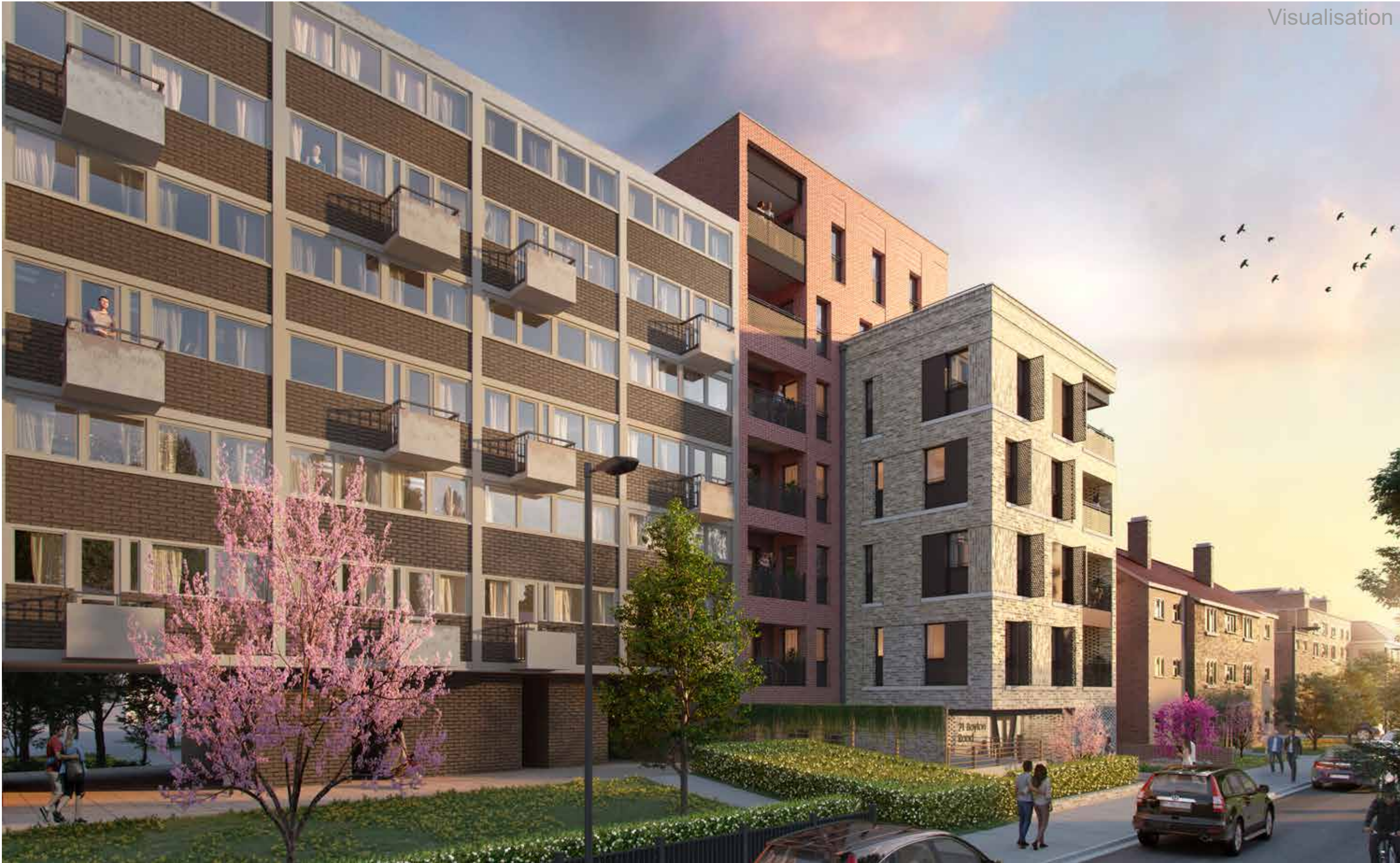
Street view looking South-East on Boyton Road
