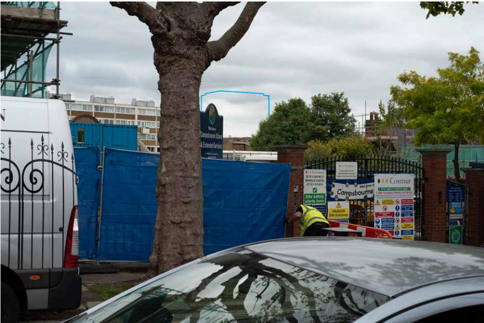
VP03. From Nightingale Lane adjacent to Campsbourne School entrance gate. Wat Tyler House is clearly visible to in the distance beyond the school playground and the proposed building will extend the visible built form to the south. Wat Tyler House has marked visual impact on this eastern edge of the conservation area however in this context the additional impact of the proposed will be limited.
