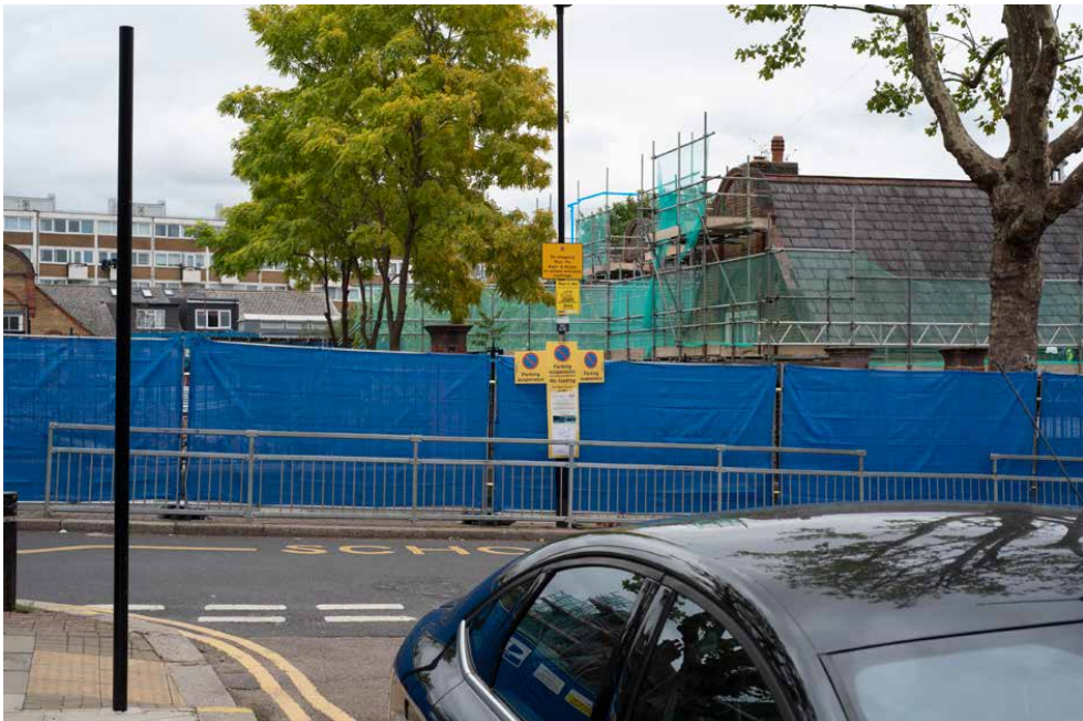
VP05. From South View Road north side. A very small part of the proposed building will be visible adjacent to Wat Tyler House. The existing school buildings and trees within the grounds largely screen the proposed. It will have very limited visual impact.
