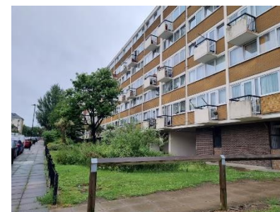
Photograph 8 West facing facade of building 1. Categorised as providing low potential to support roosting bats.
