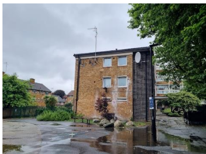
Photograph 13 Facade of east side of building 2. Categorised as having low potential to support roosting bats
