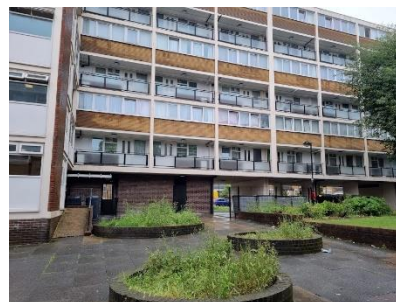
Photograph 11 Facade of east side of building 1. Categorised as having low potential to support roosting bats
