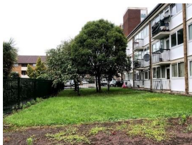
Photograph 14 Facade of south side of building 2, and group of deciduous trees including late cotoneaster. Building and trees both categorised as having low potential to support roosting bats
