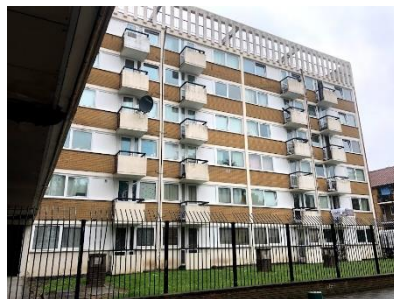
Photograph 10 Facade of south east corner of building 1. Categorised as having low potential to support roosting bats
