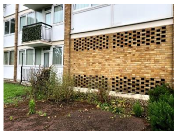
Photograph 2 Decorative brickwork on south side of building 2. Categorised as providing low potential to support roosting bats
