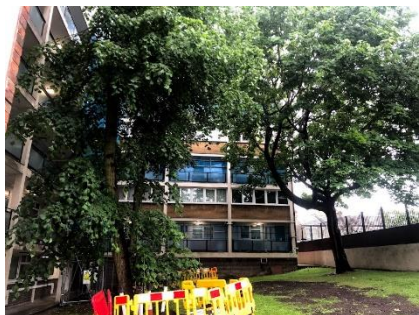
Photograph 9 North east corner of building 1, with deciduous trees on an area of amenity grassland. Trees and building were both categorised as having low potential to support roosting bats.
